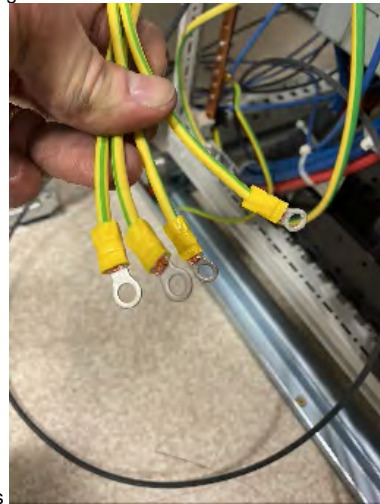
and crimped with shoes
