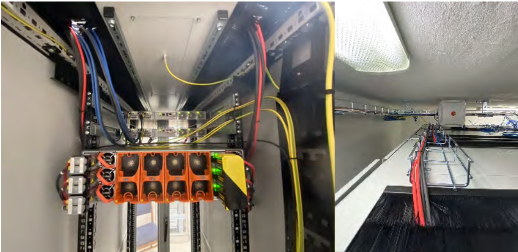
The MX2010 was connected with 5 x 63A but only 2 of the feeds were used for the new mx10003
