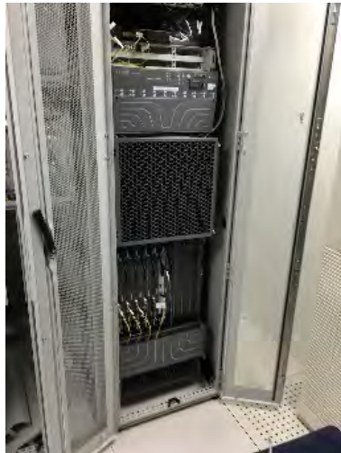
A larger site where we have three racks., 120cm deep compared to 100cm on the other core sites. The idea was that we should have the ability to place servers on four sites, Stockholm Göteborg Malmö and Luleå. So far we only have servers in Stockholm and Luleå. We also have dual AC 230V power feeds two that extra rack.
